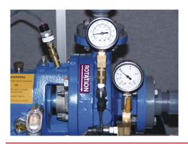
Process pumps need gauges installed, otherwise the operator has no reference point to determine the system's health.
